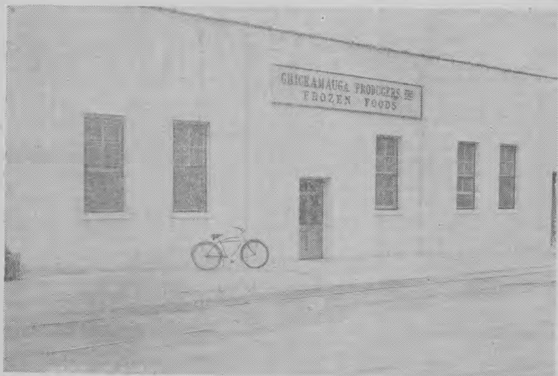
Front view of home office and storage plant, Chickamauga Producers, Inc., Cleveland, Tennessee. Here 600 lockers preserve food in frozen state for its patrons.
